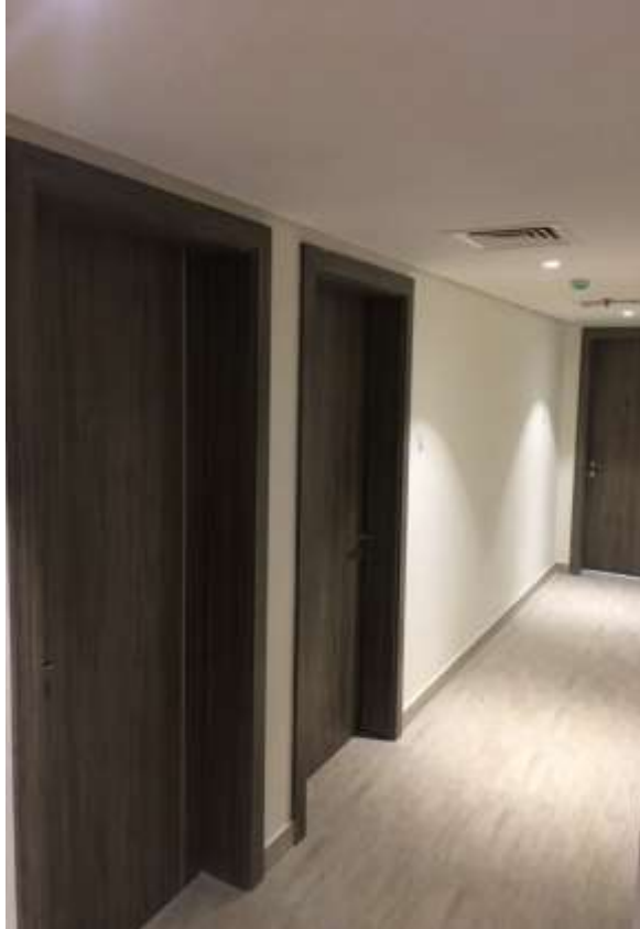
Purpose Made Doors Wooden Doors Laminate Finish
